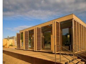
Kinetic shutters allow for shade in summer and solar gain in winter
