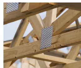
Standard gang nailed trusses must not be visible from the exterior
